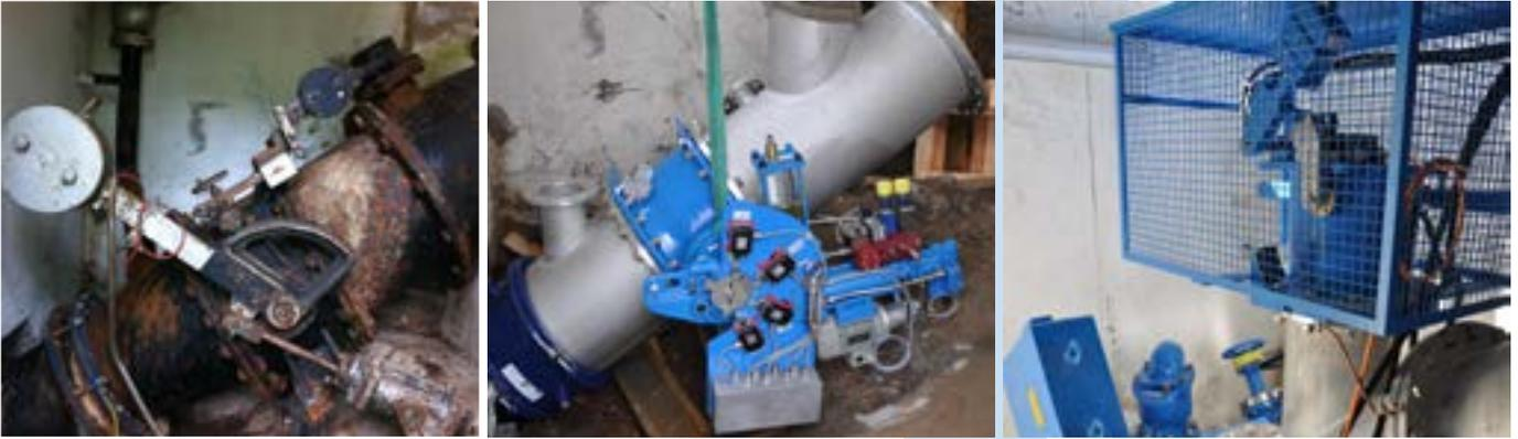
*The old pipe fracture safety device DN 600 (left) was installed in the power station in around 1965. In 2013, almost 50 years after installation, the new pipe fracture safety device (centre) was put into operation. In addition, an overspeed detector with protective cage was installed (right).*
